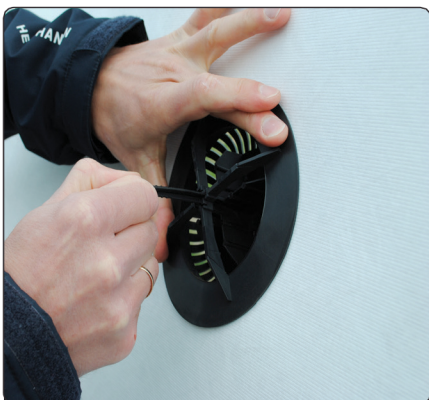
Press the underpart against the underlay, pull the strip to tighten, and lock in place
