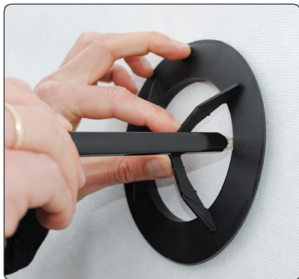
Mark and cut a hole in the underlay
